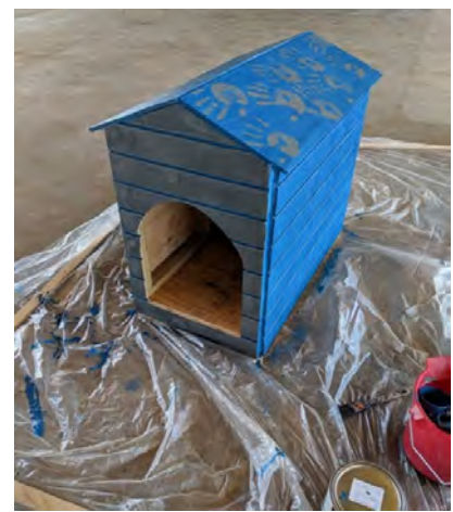
Completed doghouse construction project - USAF Scott AFB Camp -
