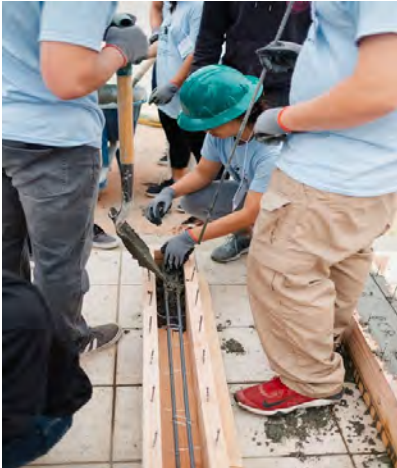
Constructing a concrete beam - US Navy Camp -
